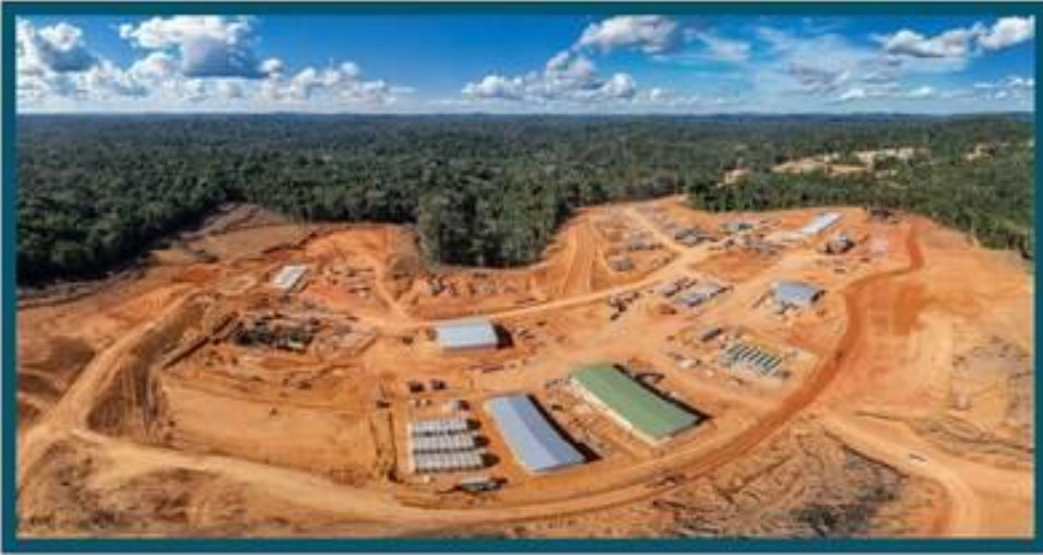
Figure 1 – Mine Infrastructure Area and Process Plant Progress
